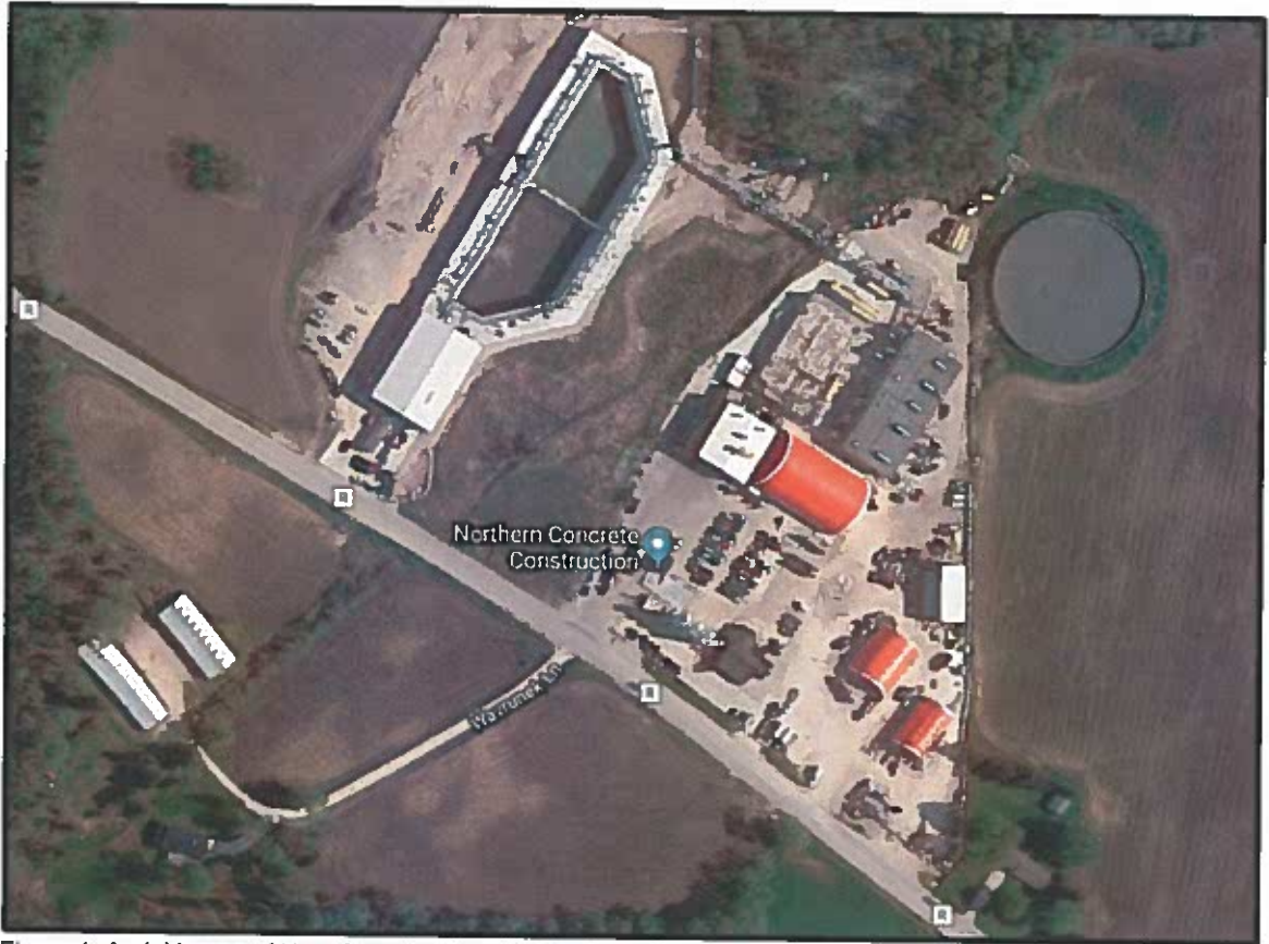
Figure 1: Aerial image of New Organic Digestion/Northern Concrete on CTH R
