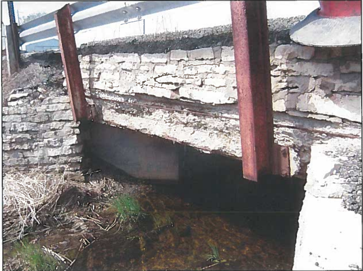
Old CTH Z structure by Fairview Road.
