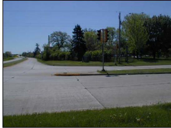
Signalized intersection at Riverside Drive and the STH 172 eastbound access road
