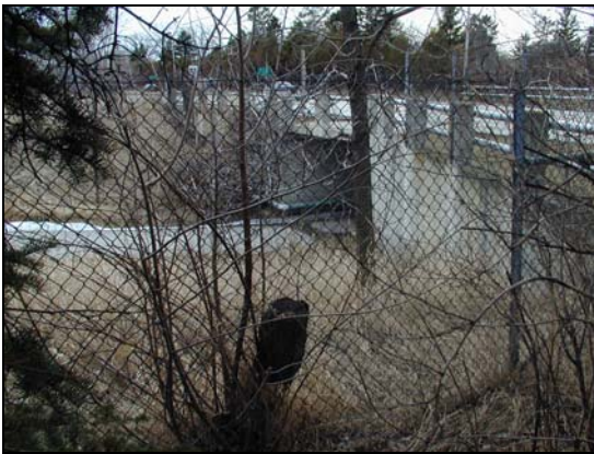
Riverside Drive underpass
