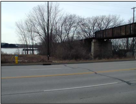
Southwest bank of the railroad trestle
