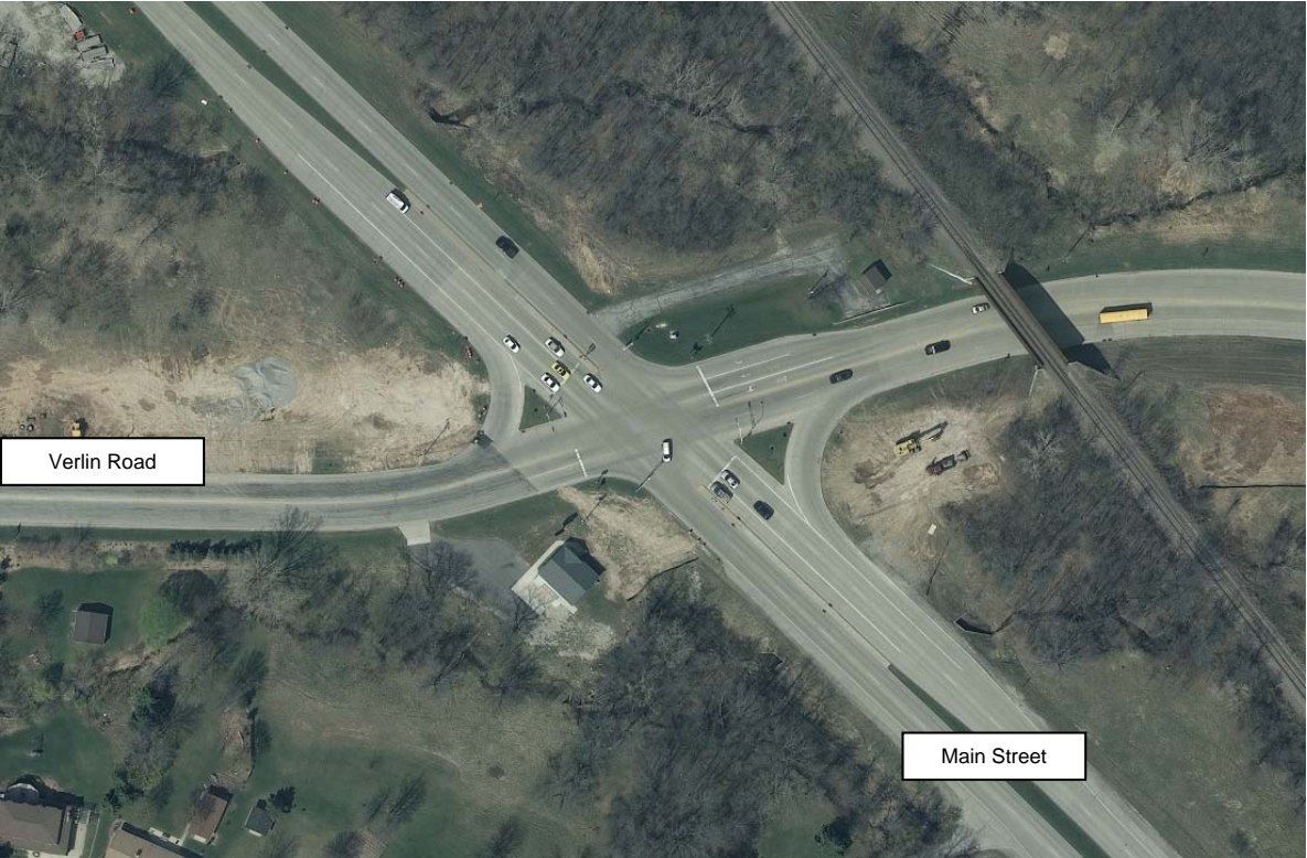
Aerial View of the Main Street – Verlin Road Intersection Before the Roundabout Project
