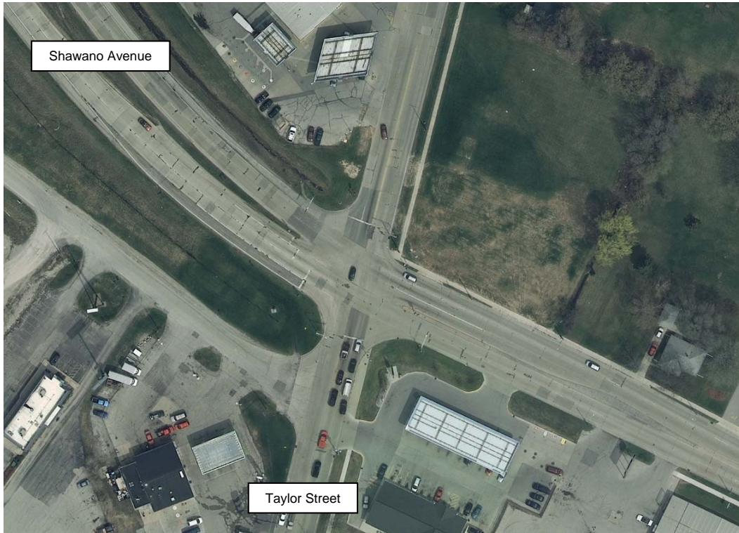
Aerial View of the Shawano Avenue – Taylor Street Intersection Before Roundabout Construction
