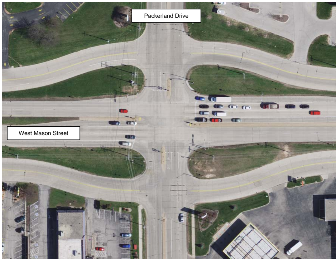
Aerial View of the West Mason Street – Packerland Drive Intersection
