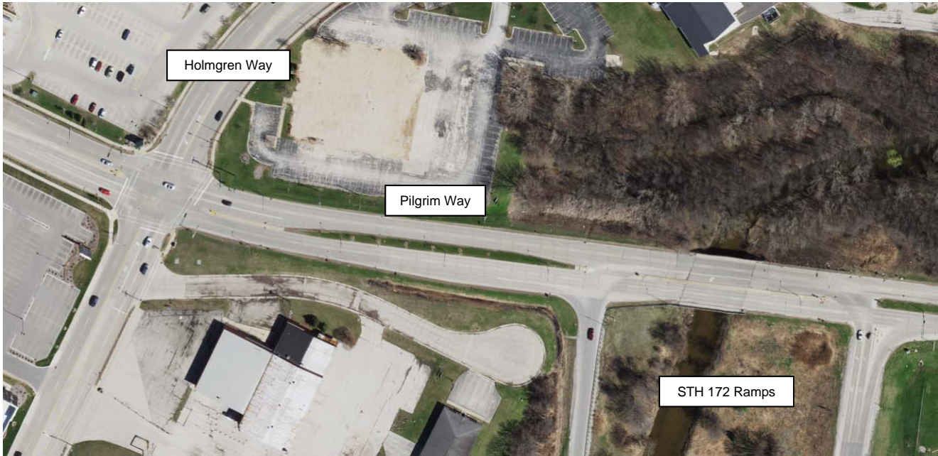
Aerial View of the Holmgren Way – Pilgrim Way Intersection (With STH 172 Ramps)
