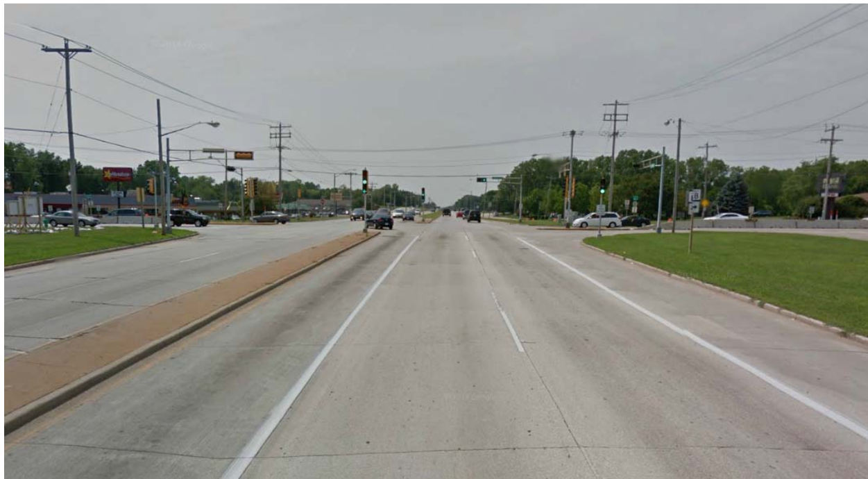
View of the West Mason – Packerland Intersection from the Westbound Travel Lanes (Picture Includes Barriers at the Frontage Road Intersections)
