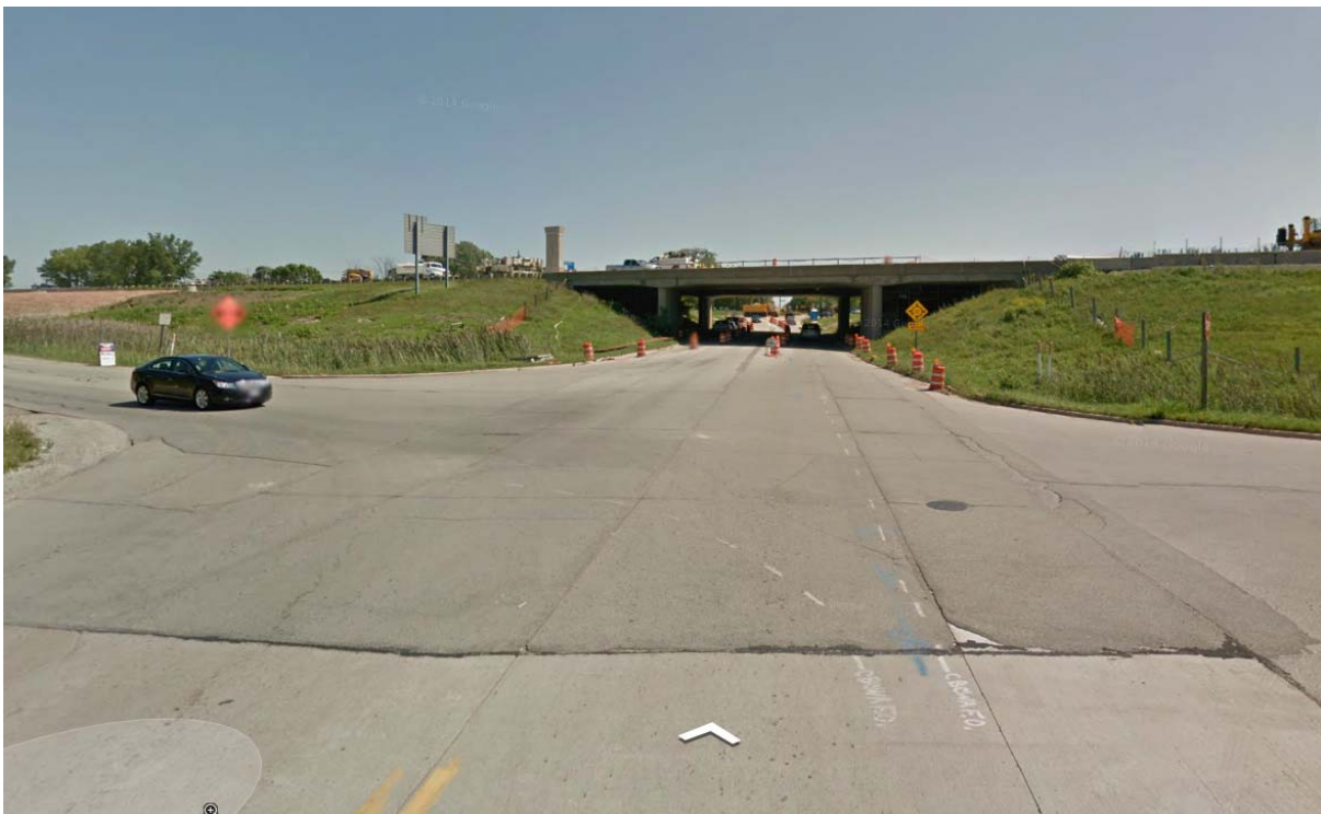
View of the US 41 Underpass from the Grant-Mid Valley Intersection
