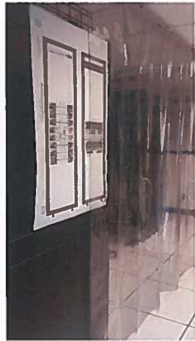
w/ Temperature Control Sheeting
