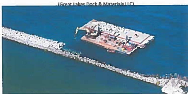
FIGURE 12 BREAKWATER CONSTRUCTION IN PENTWATER MI
