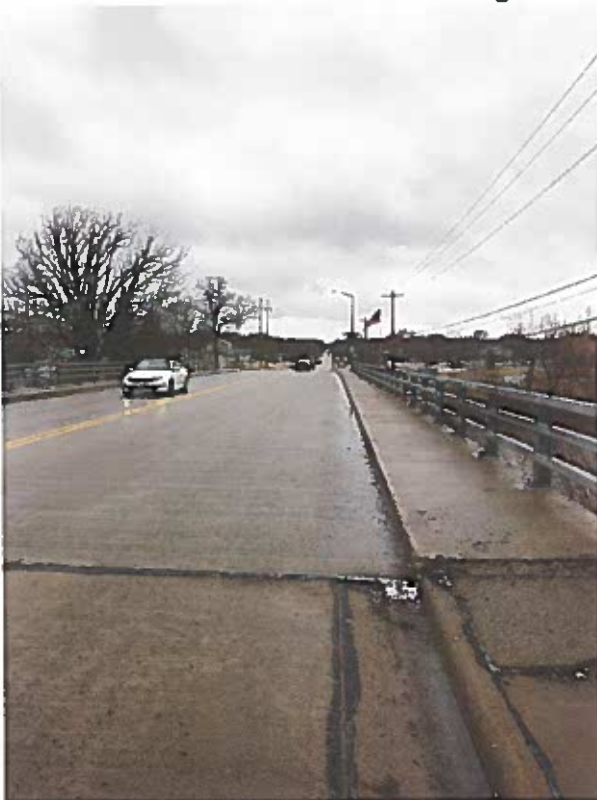
View from the bridge looking west
