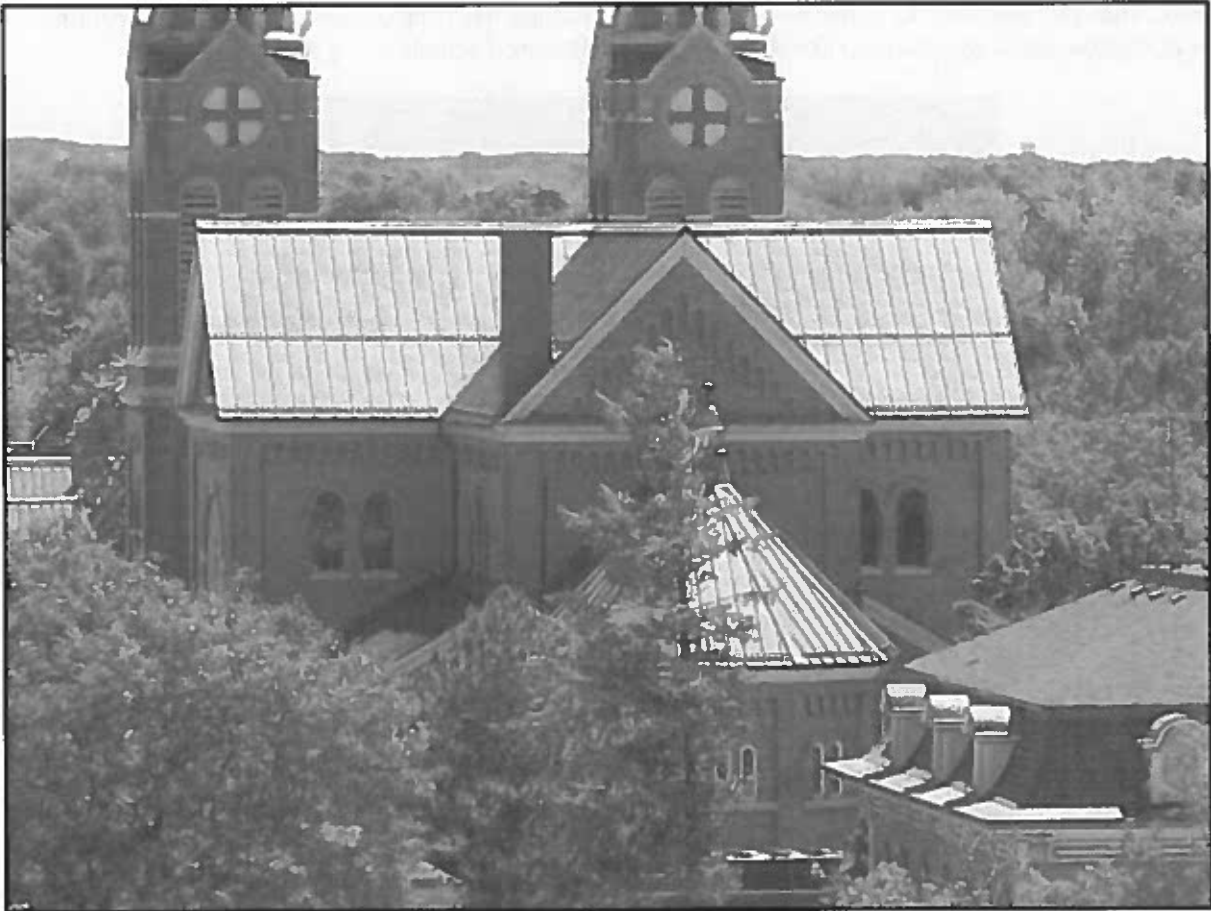
Below is another picture of the roof taken 7/16/18.
