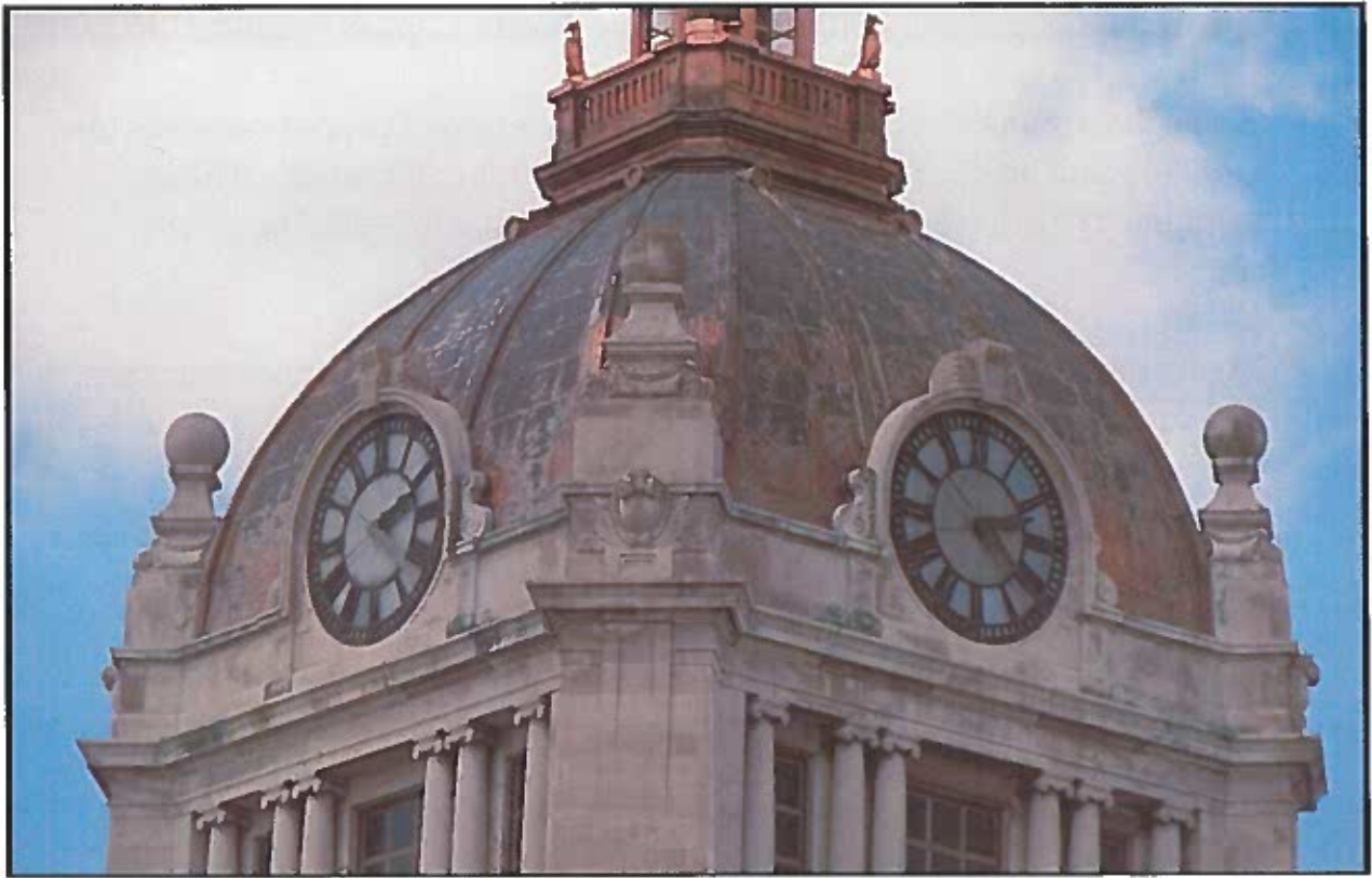
Before Restoration Project ~ 2016
