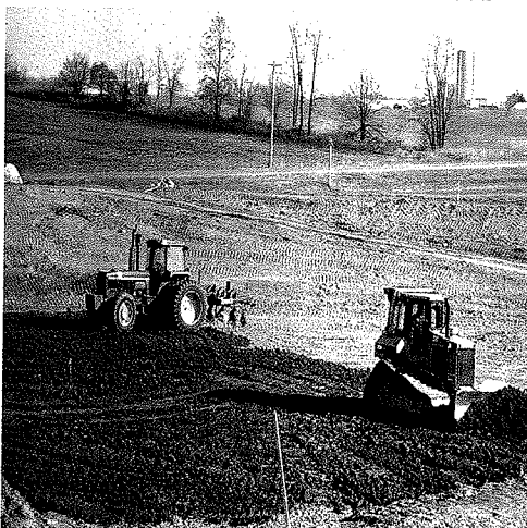
CLAY LINER INSTALLED
